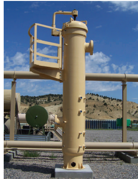
Shown above: A Type 140 Gas-liquid Coalescer ready for installation at a major gas producer in Colorado.
